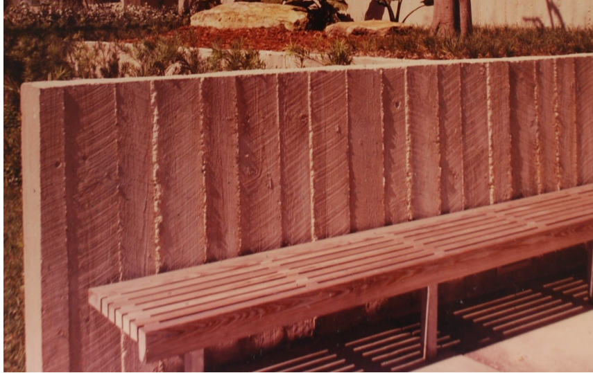
Detail showing Lapidus' use of concrete. While concrete was principally employed for its durability, Lapidus also used concrete in his designs for its texture which he believed created visual excitement.
